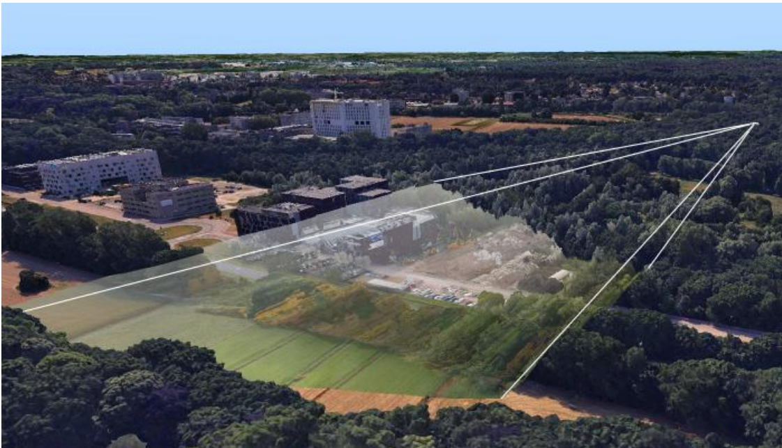
Figure 2 An illustration of video footage of our Leuven office area visualized in LuciadRIA
