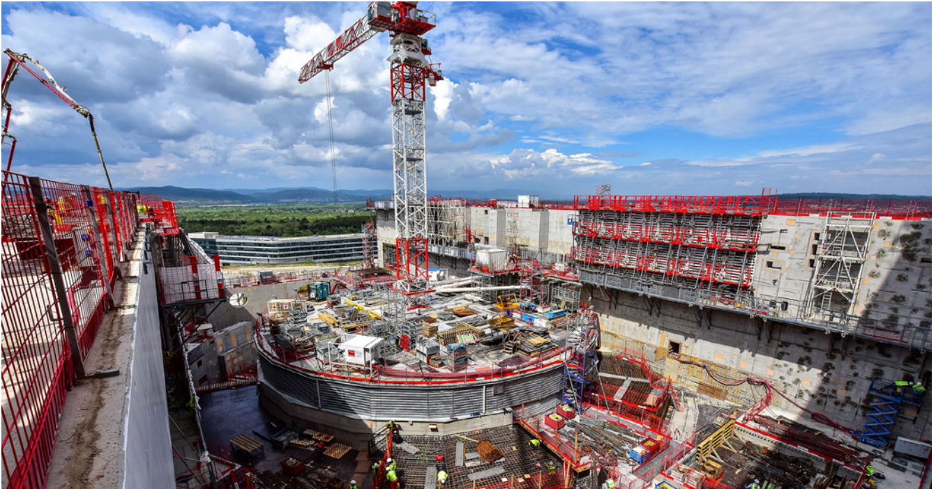
The tallest concrete of the Tokamak Building offers a spectacular and unusual viewpoint for works underway around the central Tokamak pit at the ITER construction site. © F4E
