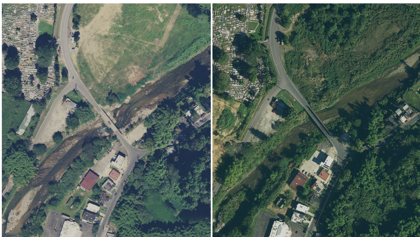
Figure 2. Aerial imagery of a bridge over the Guaonica River in Utuado, Puerto Rico, in 2017 (left) and 2022 (right). (Source: Hexagon)
