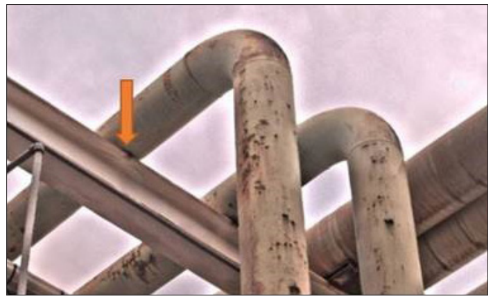
Figure 1: (Top) A model of a typical wide-flange structural beam supporting a pipe in CADWorx, which can be used to generate both the CAESAR II and GT STRUDL models. The beam needs to be designed to support pipe loads such as pipe dead load, content load, thermal load, wind load, etc. (Bottom) Site photograph of the piping and structural system.
